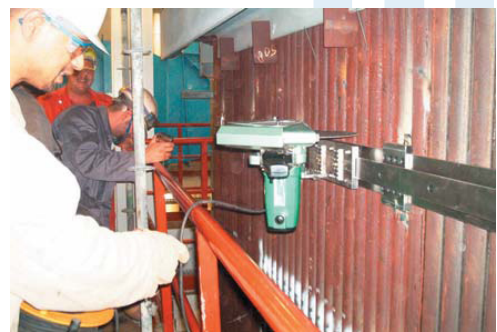
Boiler wall cutting
